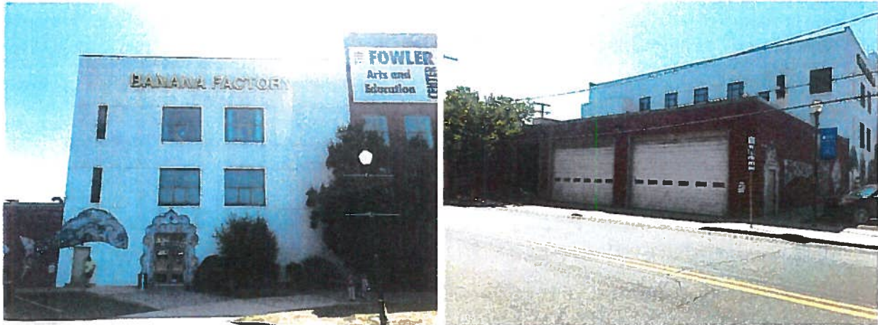
Left: Parking lot elevation (western exposure), Right: 2 nd Street elevation (northern exposure)
